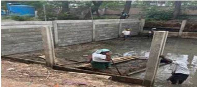
Geotextile Layer Installation and Precast Pole Installation Progress: Marking and arrangement of Pre-Cast Panels
